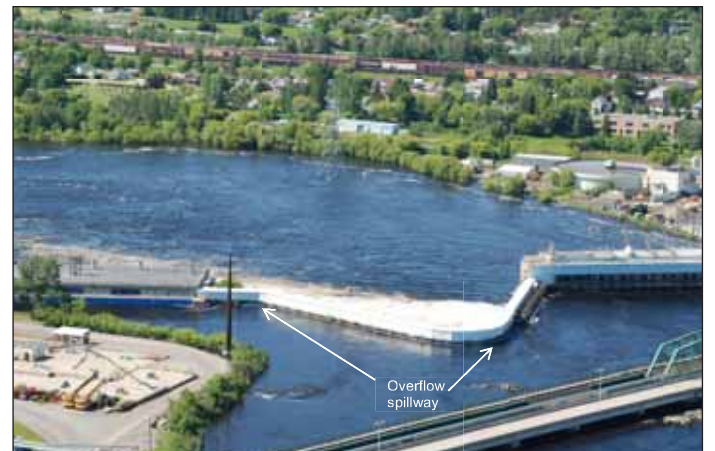
A broad view of the spillway shows the lay of the land in Fort Frances where the Rainy River begins.
