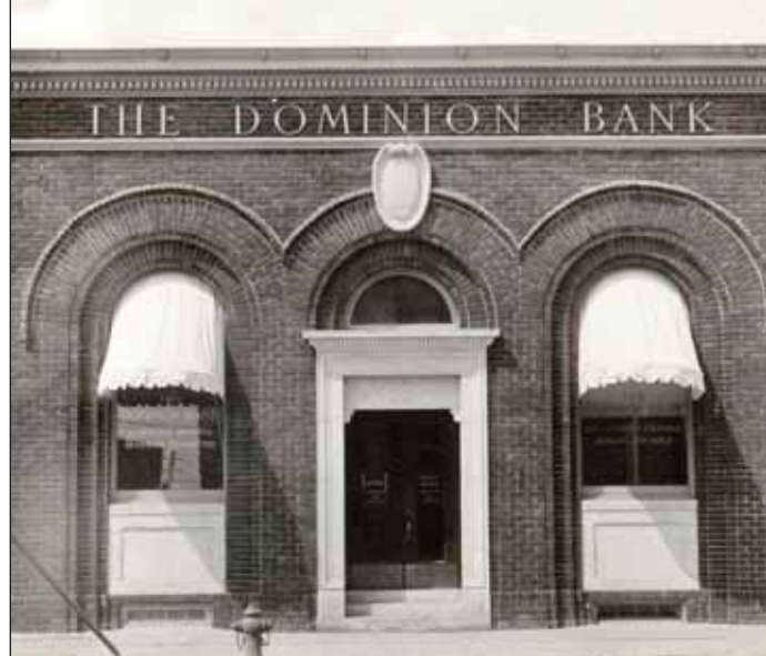
The Dominion Bank erects a new building at its current location on the corner of Scott and Mowat on February 8, 1922.
