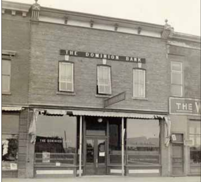
The Dominion Bank opened its doors June 20, 1914 at 232 Scott Street.
