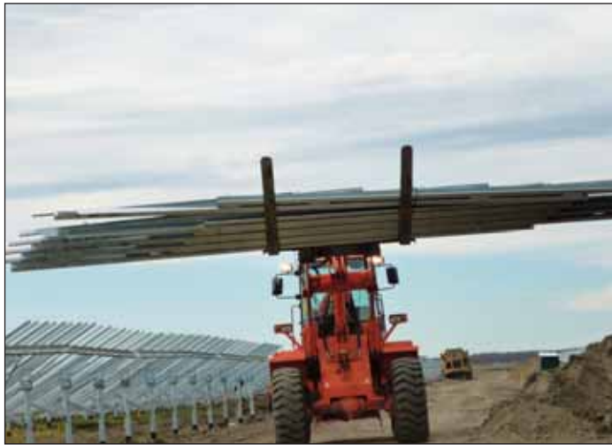
Over 800 truckloads of equipment were delivered to the sites.
